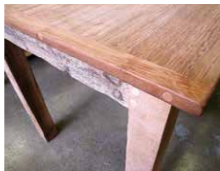
A breadboard attached with pegs
